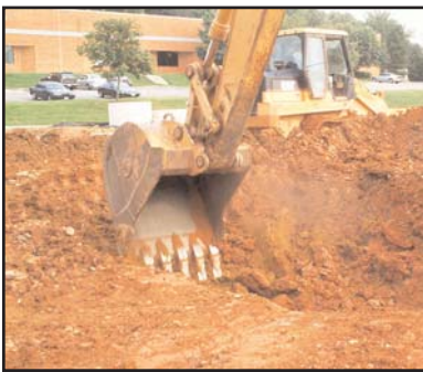
Excavate to solid subgrade.
