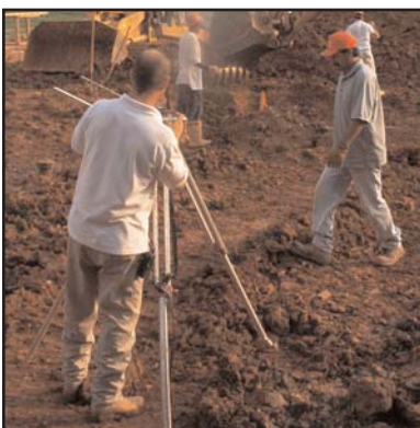
Verify subgrade elevation. Adjust base as needed.
